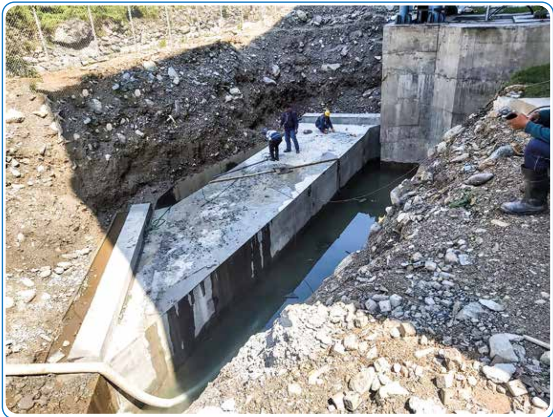
U#1 Tailrace culvert outer part of Mistri Khola HEP
