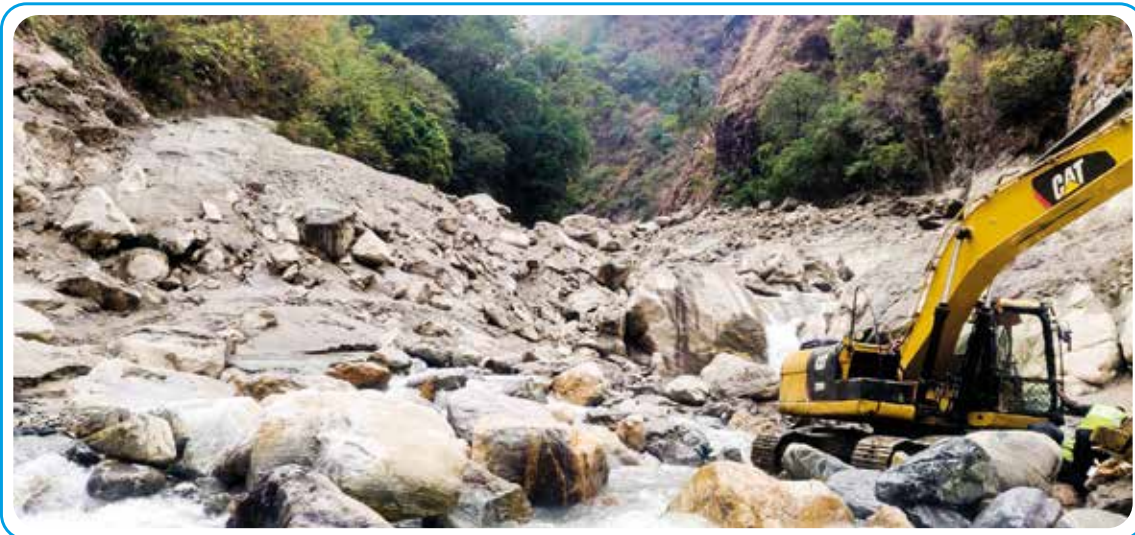
River diversion during sill beam work-at dam of Mistri Khola HEP
