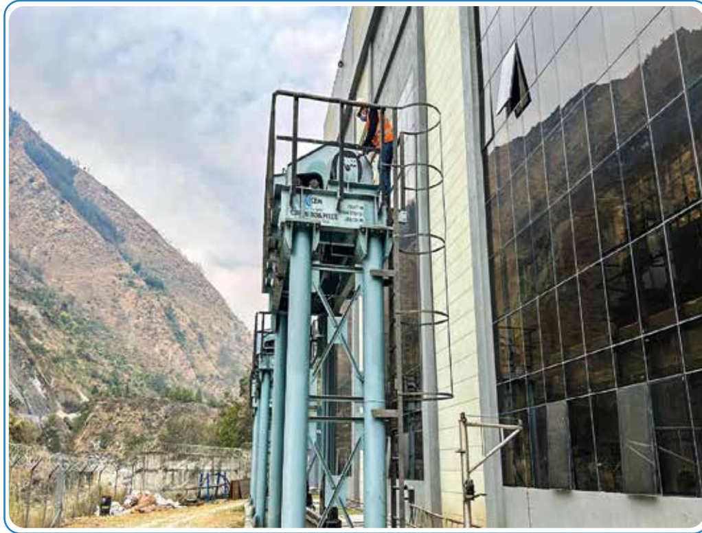
Monthly Inspection of tailrace gates of Mistri Khola HEP
