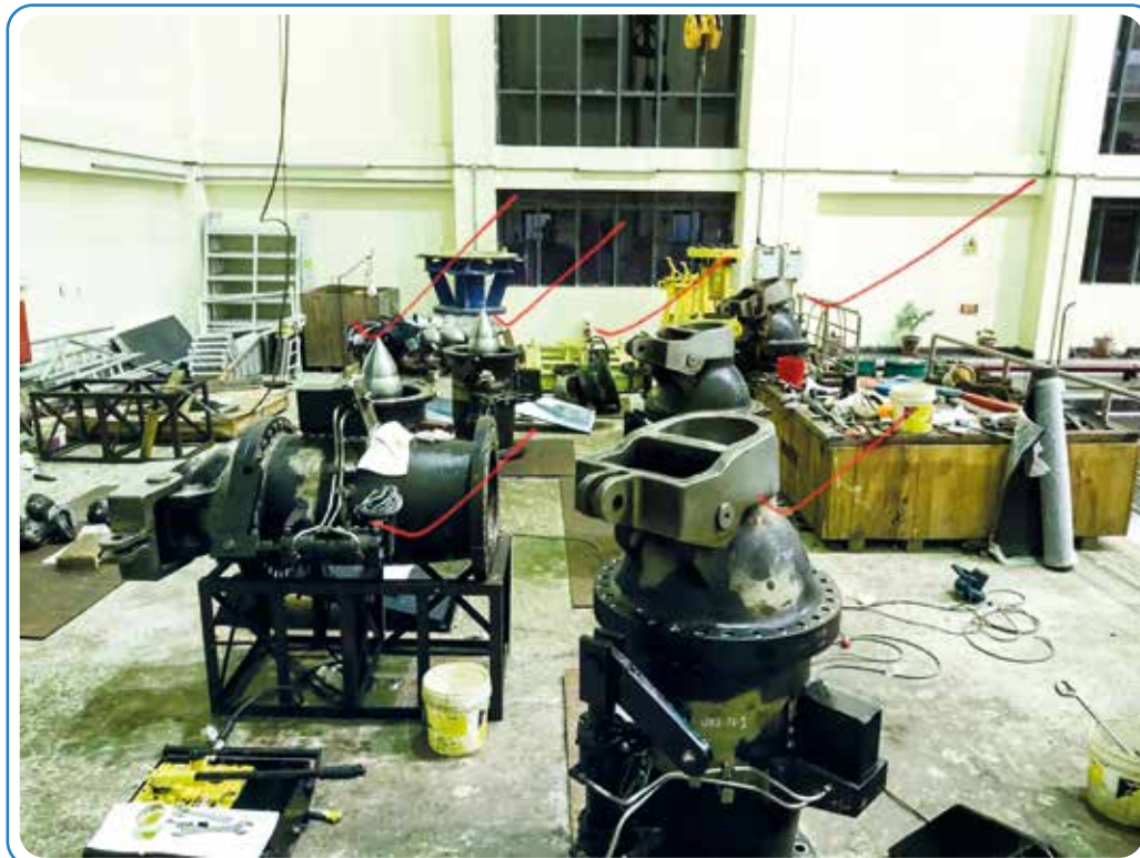
Nozzle overhauling in Unit#2, 2080 Magh of Mistri Khola HEP
