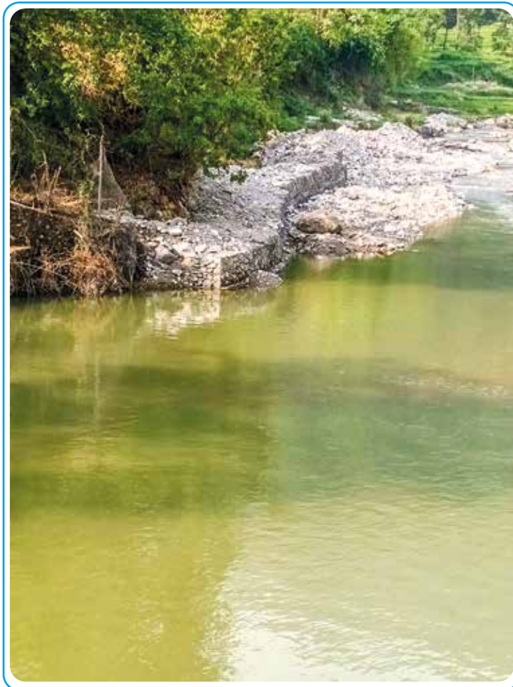
Protection Wall for Headworks of Tadi Khola HEP
